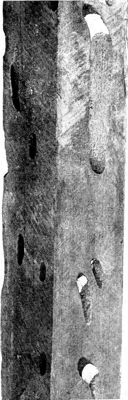
FIG. 210.—Säl house-post, showing galleries and pupal chambers of Eolesthes holosericea , Fabr., in the wood. Garhwal, January 1907.
